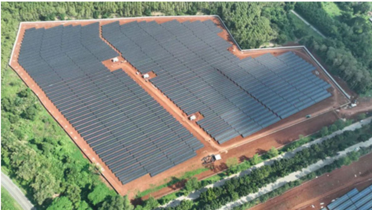
Karawang ground-mounted PV project in Indonesia
