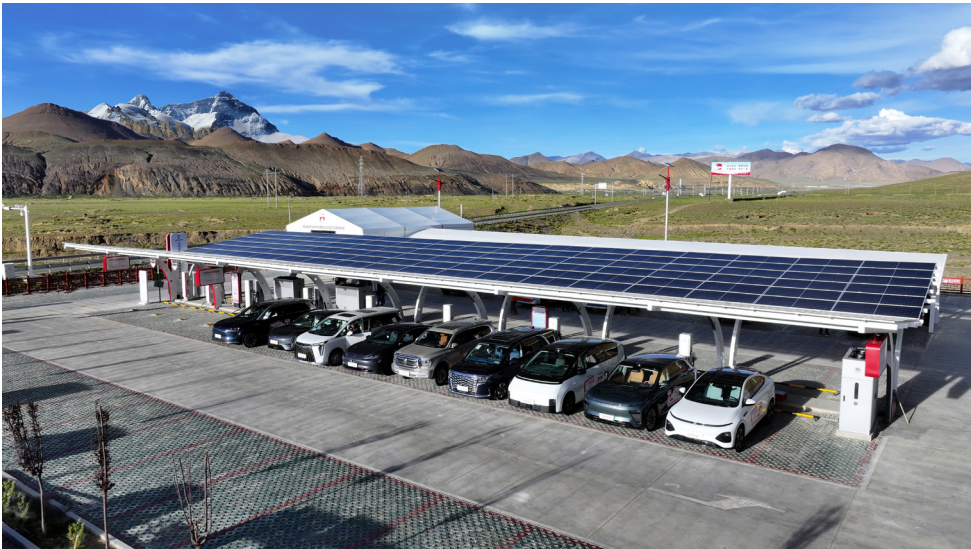
Liquid-cooled ultra-fast charging station equipped with PV+ESS at Mount Qomolangma
