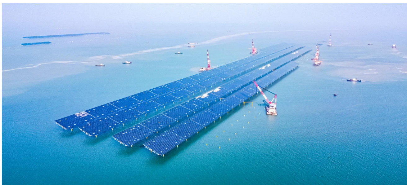
HG14 offshore PV project
