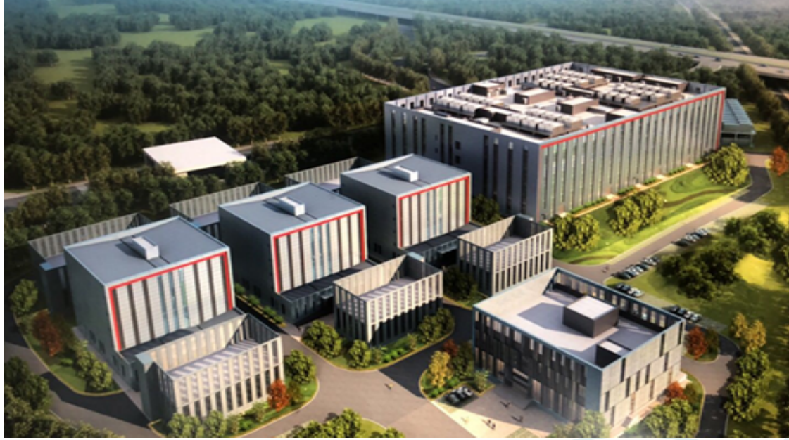
Figure 1.1. Cloud Data Center
