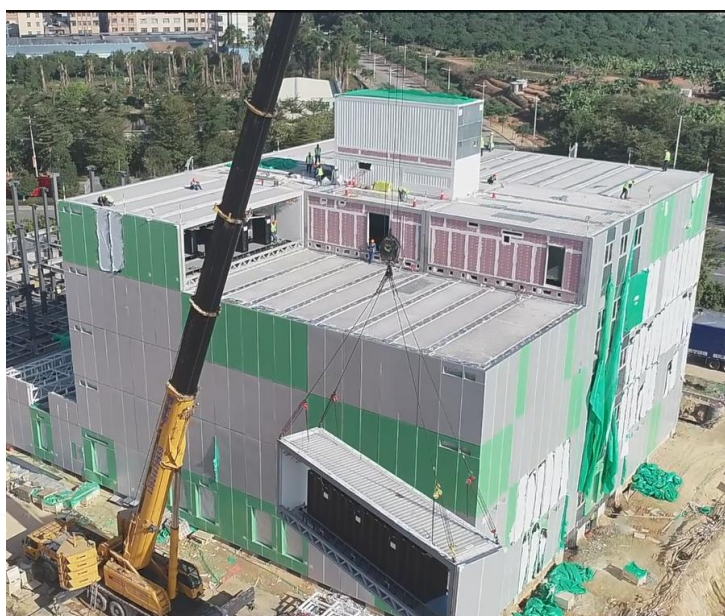
Figure 4-4 Onsite module hoisting
