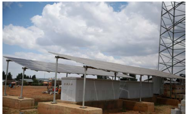
Figure 7: DG-removal by adding PV, reducing OPEX by 81%/year in Pakistan
