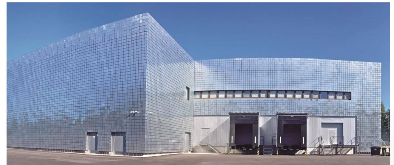
Finland - Data Center
