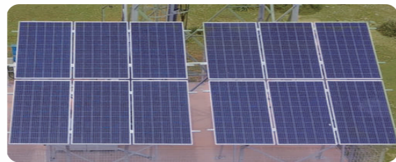
Figure: Green electricity construction for telecom sites of carriers
