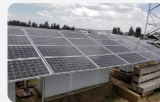
Site | Equipment room | Data center
