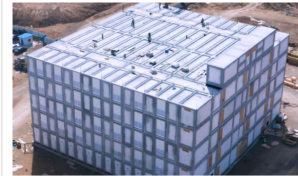
Ulanqab Huawei Cloud Data Center
